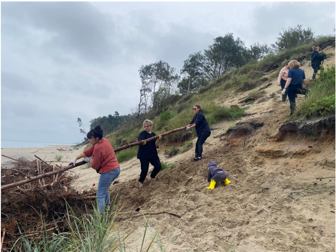
Volunteers are repairing a dune near the "Royal Forest" (Korolevsky Bor) tourist trail. March 15, 2023. Source: Curonian Spit National Park website.
