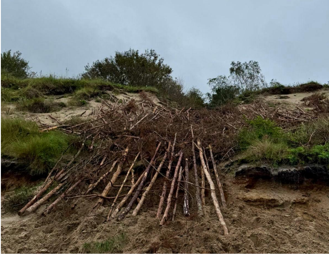
The result of volunteer work to repair the foredune near the "Korolevsky Bor" tourist trail. March 15, 2023. Source: Curonian Spit National Park website.
